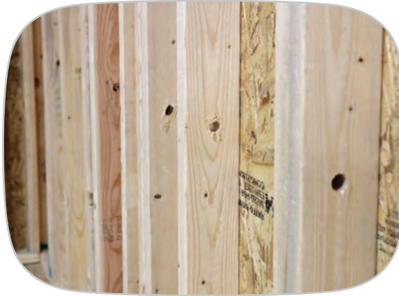
▶ 3/4" pre-drilled bore size
